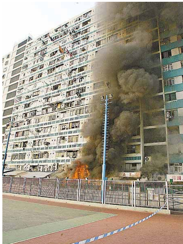
Restaurant fire due to flashover (Apple Daily, 7 January, 2005)
