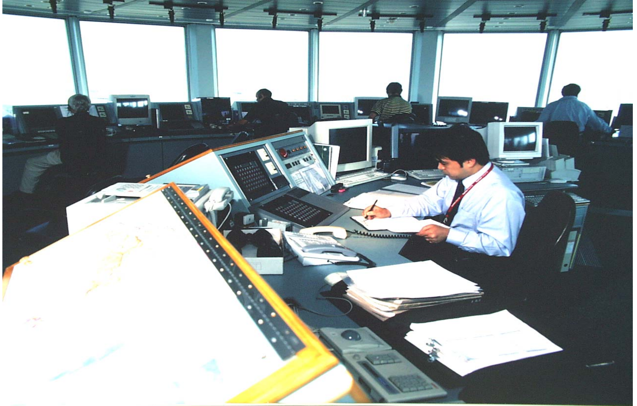
Aerodrome Control Tower
