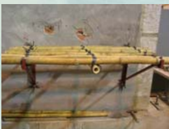
Anchored on brick
