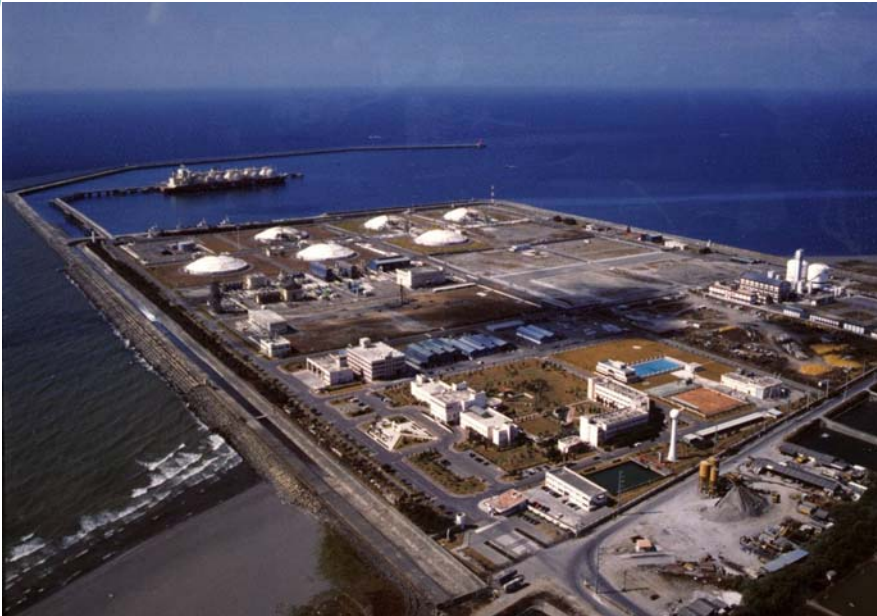
Bird's eye view of LNG plant
