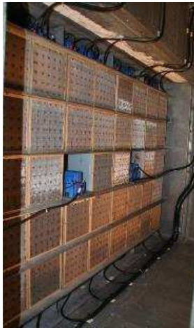
Air Disinfection Devices mounted inside the AHU
