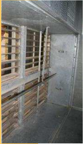
Inside of AHU before installation
